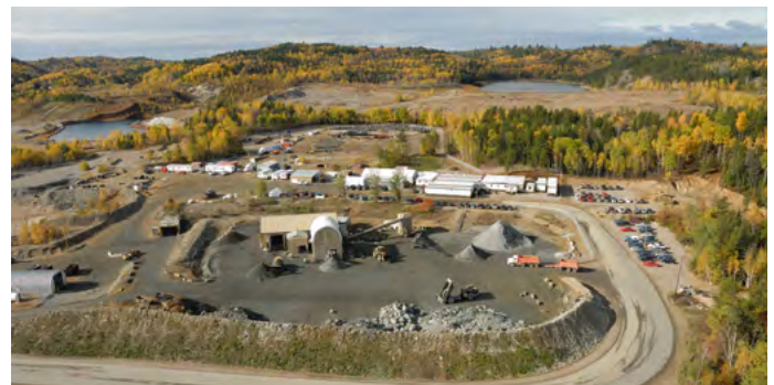
McCreedy West Mine, October 12, 2007
