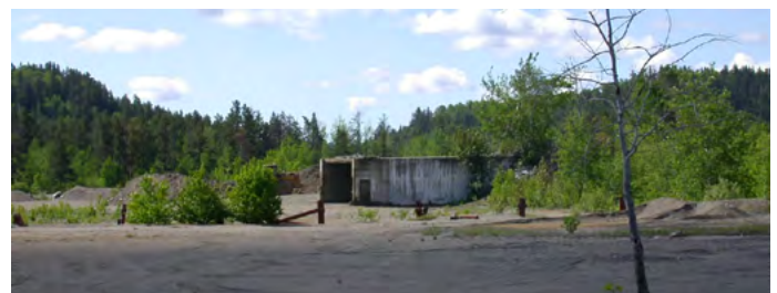
Surface concrete adit (tunnel entrance) to the McCreedy mine ramp in 2002, prior to the FNX acquisition
