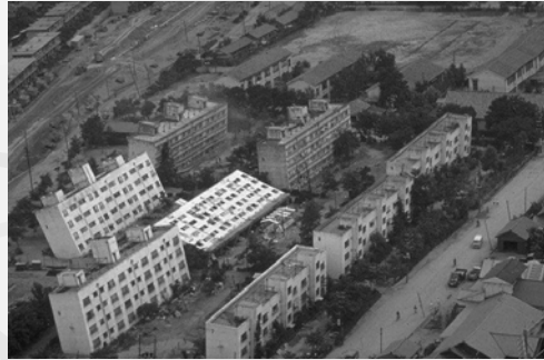
Buildings built on poorly consolidated sediment -tilted due to sediment liquefaction resulting from earthquake
