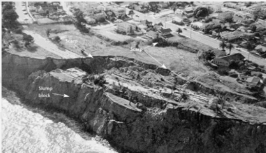
Subdivision at Point Fermin, California -shore undercut by waves, poorly consolidated material highly unstable -add seismic activity, and you're toast !
