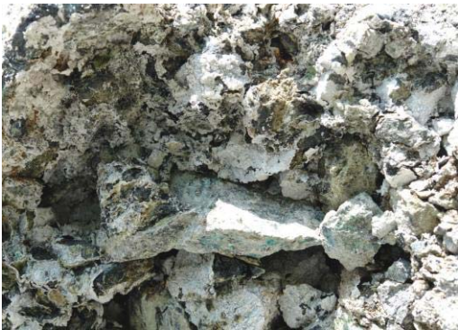
Figure 1: Example of hydromagnesite incrustation at Montecastelli
