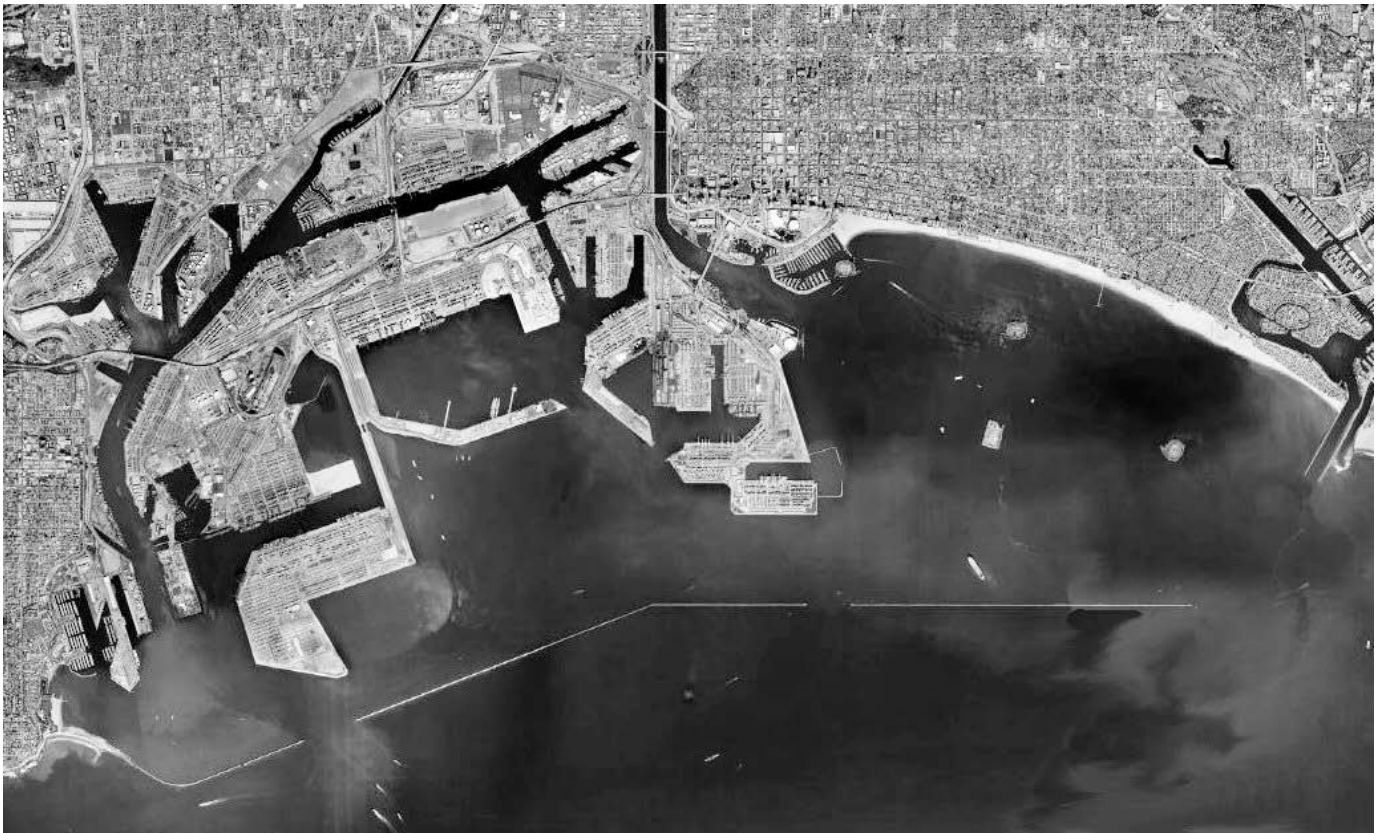
Figure 6: Port of Los Angeles/Long Beach and 8.5 mile breakwater
