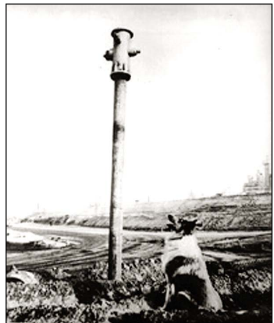
Figure 5: Subsidence-frustrated Long Beach Local
