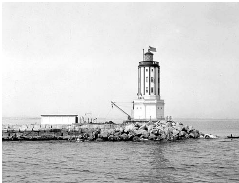
Figure 7: Angles Gate Lighthouse on the San Pedro Breakwater was built in 1913.
