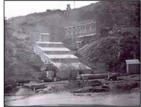
Figure 36: Ore processing plant at Wight's Cove for the Black Jack mine (circa 1925).
